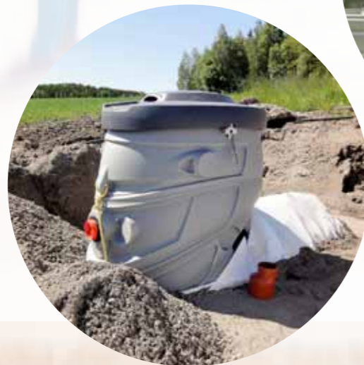
Installation of a single house treatment system
